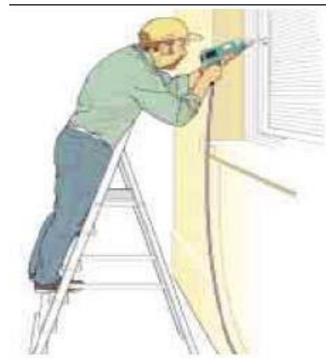
Correct – steps facing work activity
